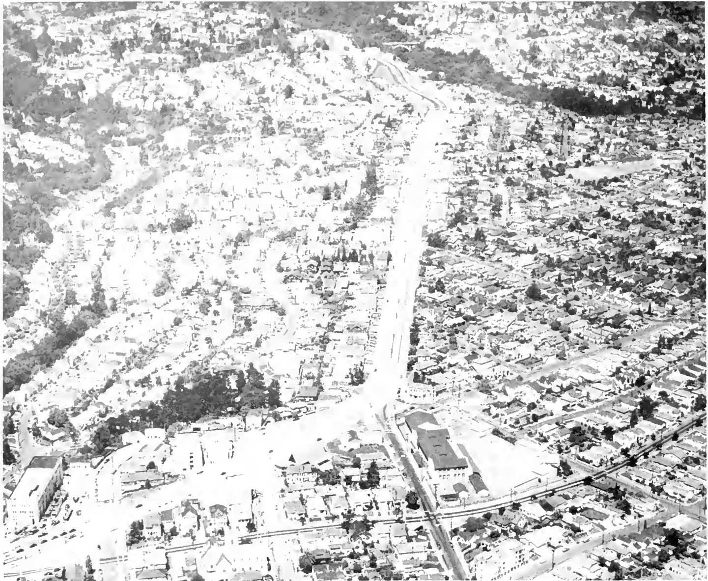
Aerial view of Park Boulevard from Excelsior Avenue to Estates Drive. Foreground shows beginning of one mile of concrete pavement; upper 0.4 mile of pavement is asphaltic concrete.
